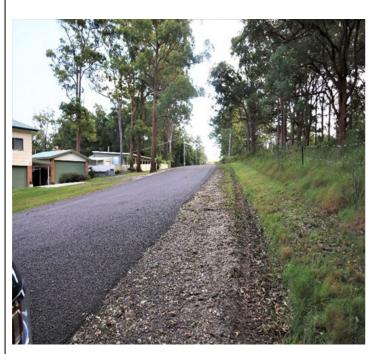
Advice from long term residents is that the Surface flooding into Merriwa Blvd. is primarily coming from this area along Gloucester St. and land north and west of this intersection. Someone has recently driven the tyres of a heavy vehicle along the verge where a good size Table Drain should be. This slight indentation would have little impact on the directional control of surface flooding during heavy rains.
