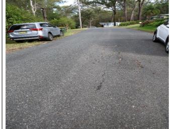
Taken during 2024 review. Road surface damage due to heavy Cross Road flooding since 2023 Review. Previous patching evident.
