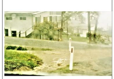
South side Table Drain in Merriwa Blvd. west remains partly shallow. North side drain is now a good size.
